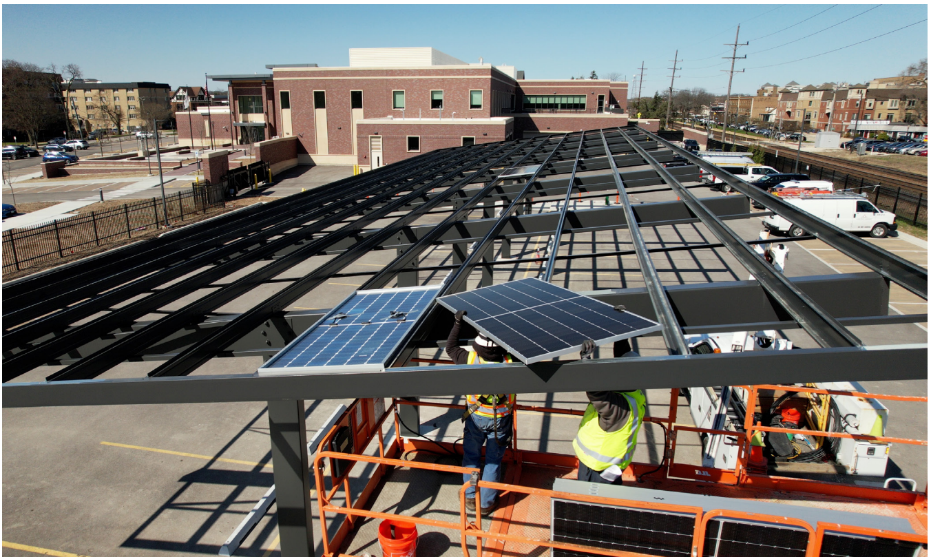
Installation of a solar car canopy at the Civic Center in April 2025. When completed, the Civic Center will have a 160 kW solar array to generate renewable electricity for the facility.
